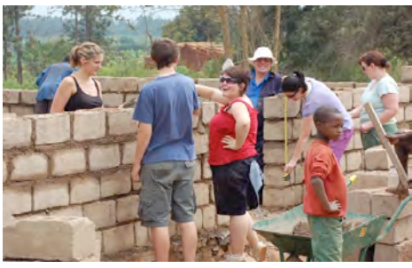
Rwanda 07 team, helping to build houses in Bugesera
