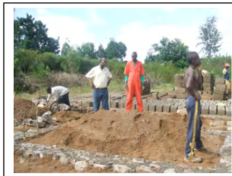
Building a House for Chantal
